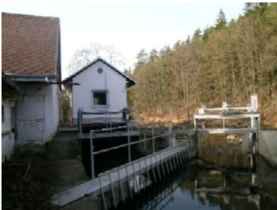
Obr. 7: Vtok do MVE, hrubé česle a jalová propust
