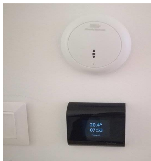
Obr. 13: Senzor CO 2 [2]
